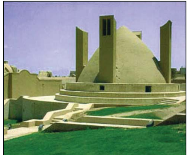
Figure 5. Cistern ventilated and cooled with windcatcher
