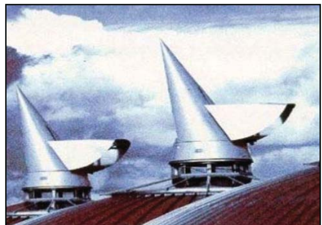
Figure 6. Windcatchers at Bluewater Shopping Center [4]
