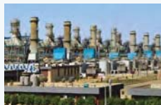
Suleymaniyah Combined Cycle Power Plant - Iraq
