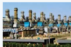
Suleymaniyah Combined Cycle Power Plant - Iraq
