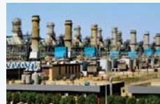
Suleymaniyah Combined Cycle Power Plant - Iraq
